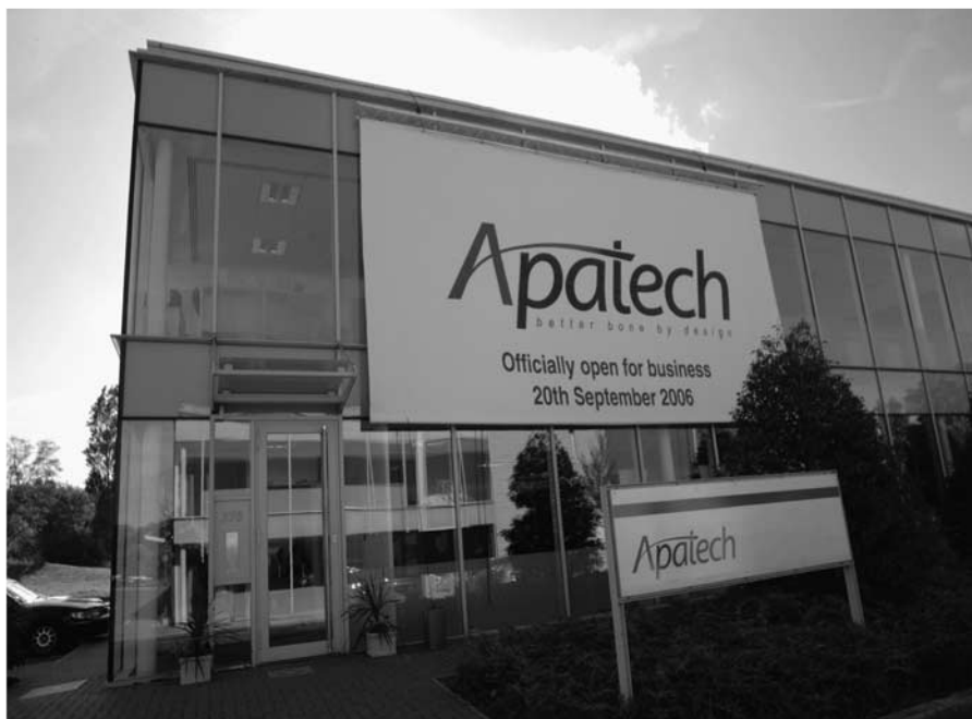
Figure 2: New ApaTech headquarters, Elstree, Middlesex, UK
