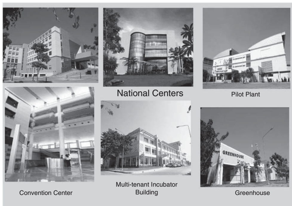
Figure 3: Infrastructures in Thailand Science Park.
